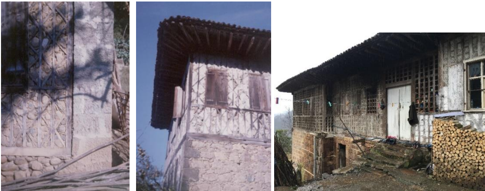
Figure 12. Stone Material Used as Filling Material and Stone Material Used in The Basement-Turkey
